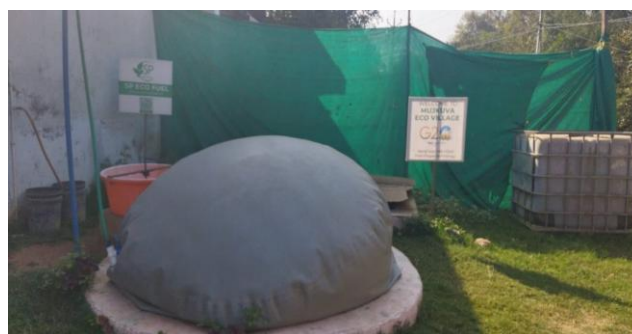
Visit to domestic biogas plants of small capacity (2 cubic metre) at Mujkua, Guujrat
